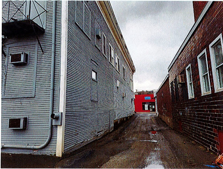
Photographs of exterior walls showing deterioration / failure of clapboards and fascia.
